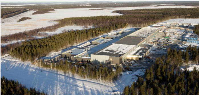
Facebook datacenter at edge of the Arctic circle ( source: CNET, 2013 )
