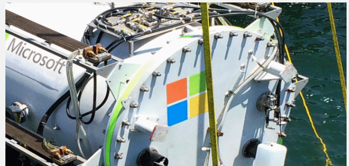
Microsoft underwater datacenter ( source: NYTimes, 2016 )
